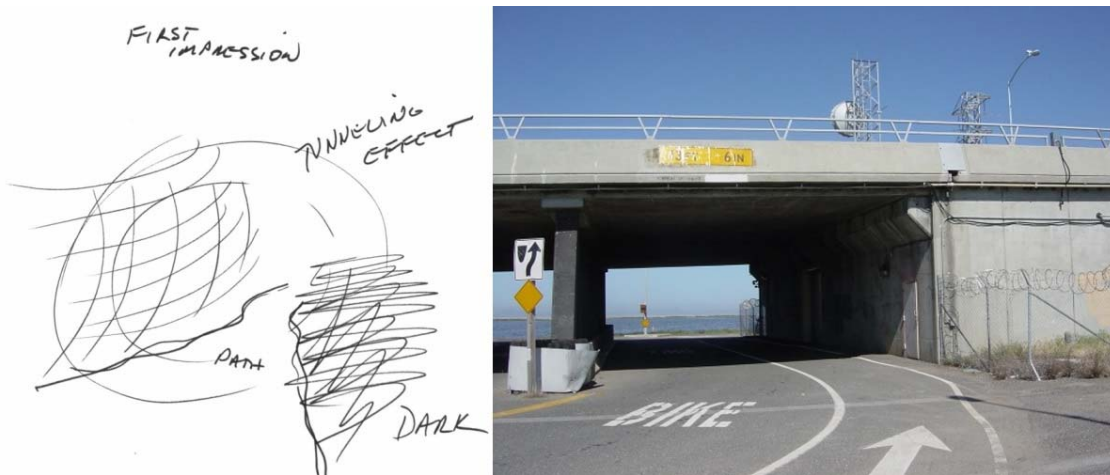
Fig. 2 Tunnel Underpass to the Site
